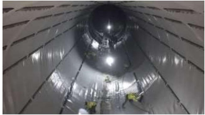
At the beginning and end of the waterproofed stretch, the SIBELON® geocomposite is fastened by a watertight perimeter seal that avoids water infiltration behind the liner
