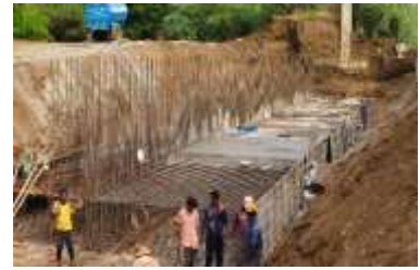
Construction of Retaining wall
