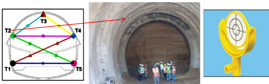
Fig. 13 : Bi-reflex targets (T1, T2,...) installed on the supporting rings
