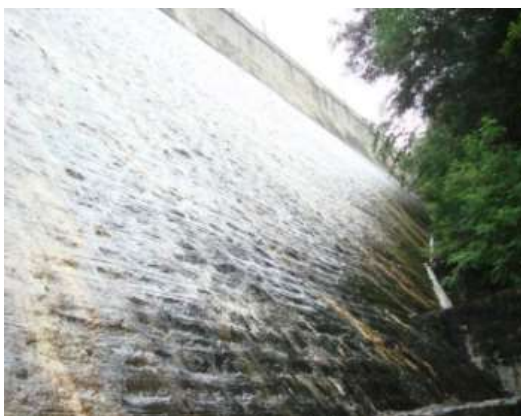
Before Geomembrane (wet downstream)
