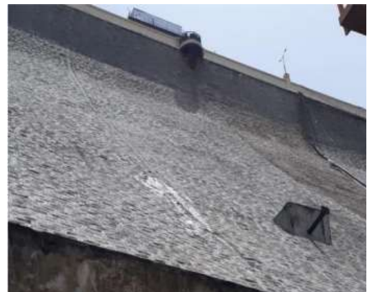
After Geomembrane (dry downstream)
