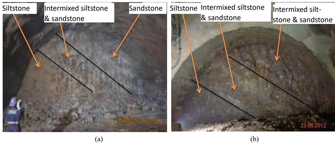
Fig. 10 : View from main tunnel, south end showing bands of various rocks of Murree formations
