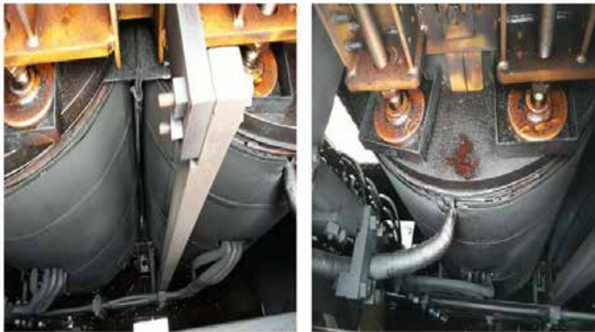
Fig. 2 : Thick Carbon Deposits Observed on the Transformer Winding Assemblies
