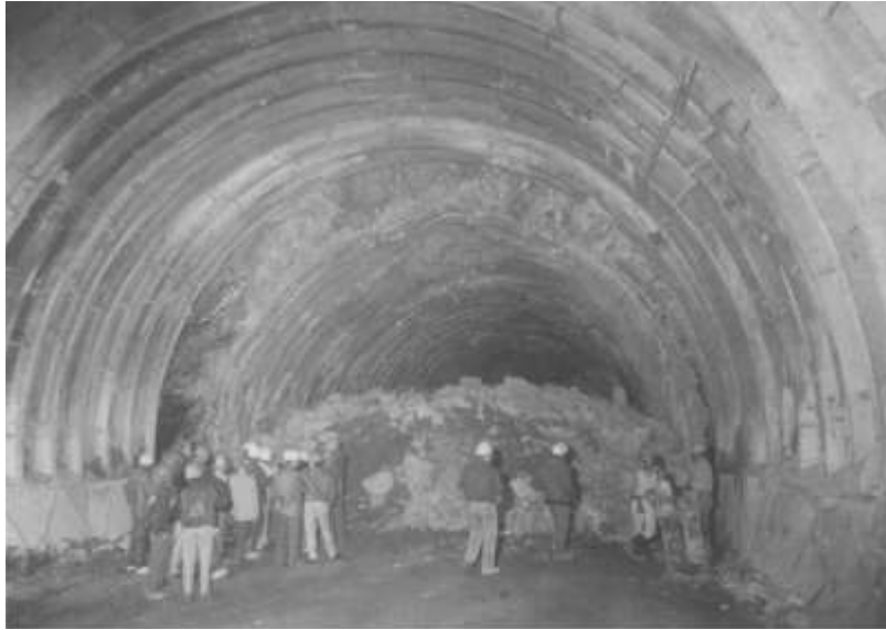
Fig. 7 : Steel ribs failed in Nathpa Jhakri HRT due to squeezing ground (Hoek, 1999)
