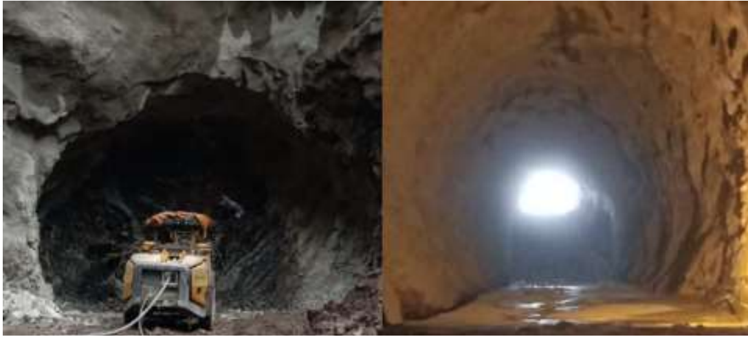
Fig. 17 : View of initial opening of inlet portal (left) and daylighting of diversion tunnel (right)
