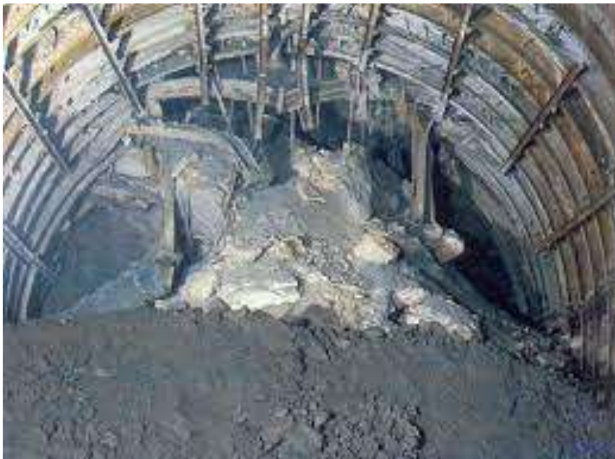
Fig. 8 : Steel ribs buckled due to squeezing ground behaviour (Dev et al., 2013)
