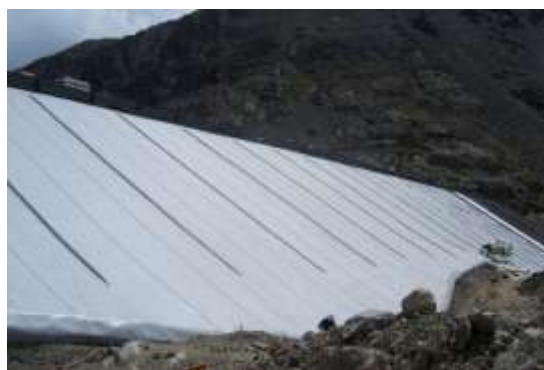
The system of tensioning profiles (left) during and (right) after completion of the installation
