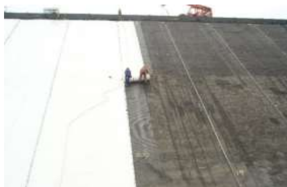
The system of tensioning profiles (left) during and (right) after completion of the installation
