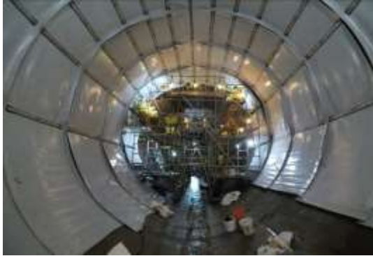
At the beginning and end of the waterproofed stretch, the SIBELON® geocomposite is fastened by a watertight perimeter seal that avoids water infiltration behind the liner
