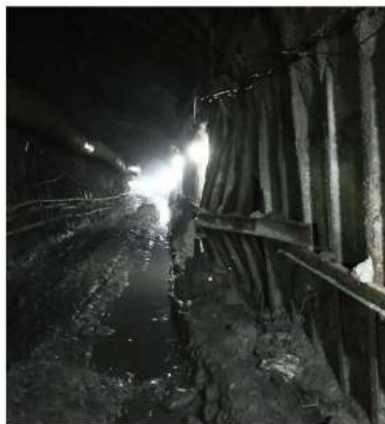
Fig. 4 : Tunnel Liner Failure - Middle Mode HRT Conditions (observed during the site visit)
