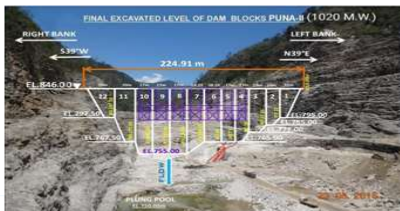
Photo 6: Final excavation level of dam blocks of PHEP-II
